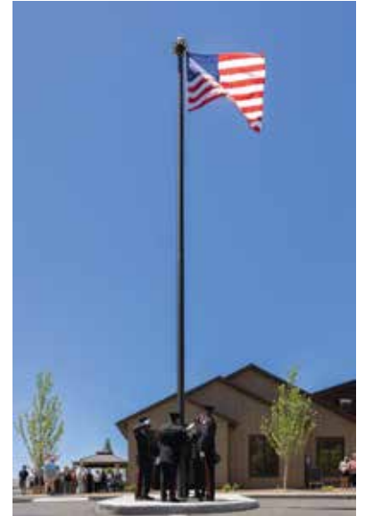
The American flag is raised over the newly rebuilt Fire Station 41 for the first time
