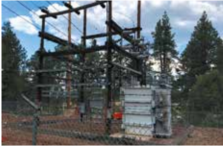
A wood structure substation served the Munds Park community prior to the substation upgrade project.
