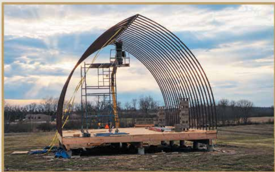
Steel shell kit during assembly
